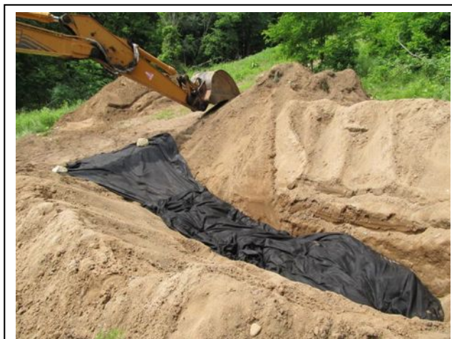
Backhoe excavates the pit, designed to maintain fairly constant temperature and humidity conditions.
