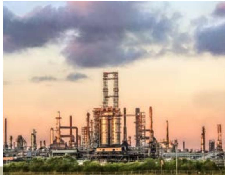
**Combined Heat and Power (CHP) system.** The refinery is constructing a state-of-the-art CHP system that will allow it to operate more efficiently while reducing greenhouse gas emissions from Minnesota's current energy supply mix. The CHP system will use natural gas and a heat recovery process to produce approximately 50 megawatts of electricity, or roughly 40% of the energy required to power the refinery. The \$150 million system is expected to be operational by 2018.
