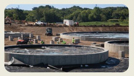
Three new ATS storage tanks are being constructed on Flint Hills Resources property at the southeast corner of Highways 52 and 55.
