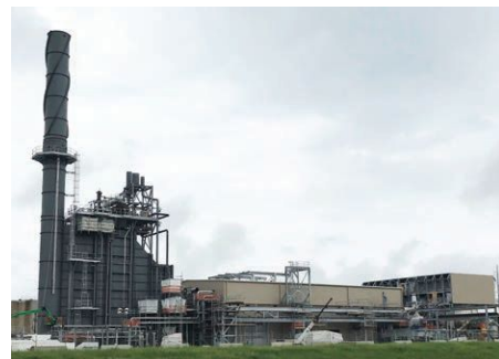
FHR's new $150 million state-of-the-art Combined Heat and Power (CHP) system will allow the Pine Bend refinery to operate more efficiently.
