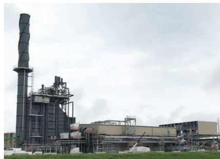
FHR's new $150 million state-of-the-art Combined Heat and Power (CHP) system will allow the Pine Bend refinery to operate more efficiently.
