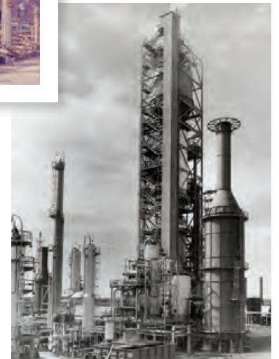
The original thermoform catalytic cracker unit
