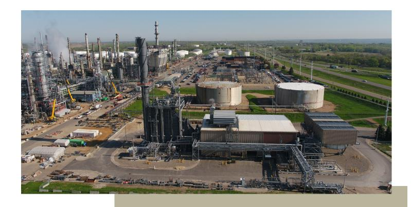
Ammonium thiosulfate technology and distribution terminal. Pine Bend's new ammonium thiosulfate (ATS) technology and distribution terminal allows the refinery to convert a traditional source of air pollution from motor fuels (sulfur) into a valuable fertilizer product that benefits farmers. One of the largest applications of ATS technology in the world, this system also helps the refinery produce ultra-low sulfur gasoline, which lowers vehicle emissions and is better for the environment.
